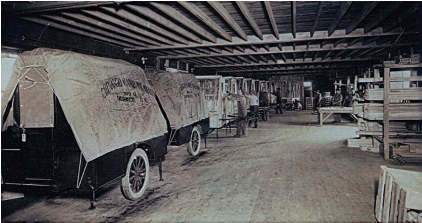
Assembly line at the Chenango Equipment Manufacturing Company in Norwich
